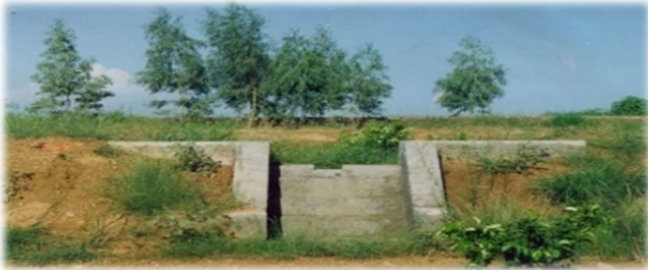
Image15: Showing concrete outlet
