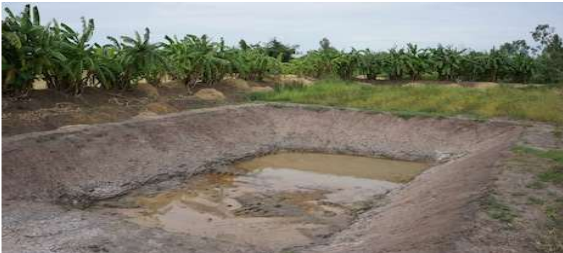
Figure 16: Earthen Bund Pond
