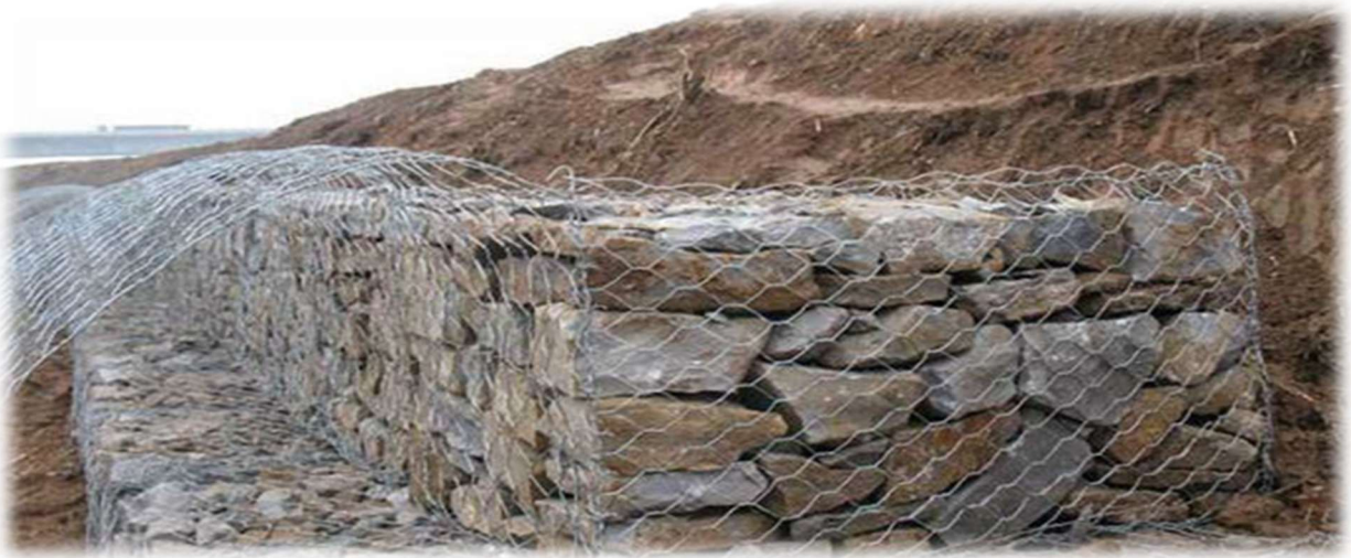
Image 12: Gabion spur
