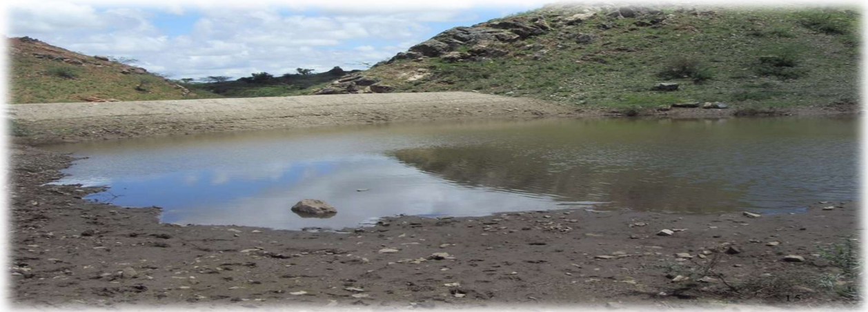
Image14: Showing earthen bund for water retention
