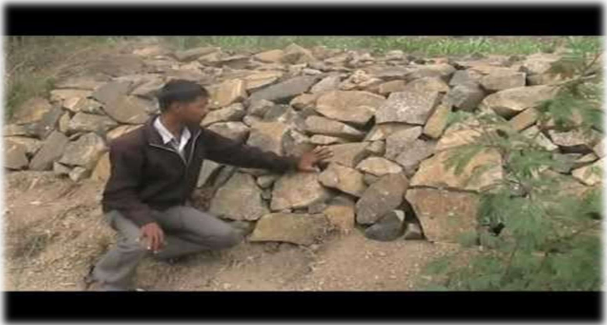
Image 11: Simple gully plugging technique
